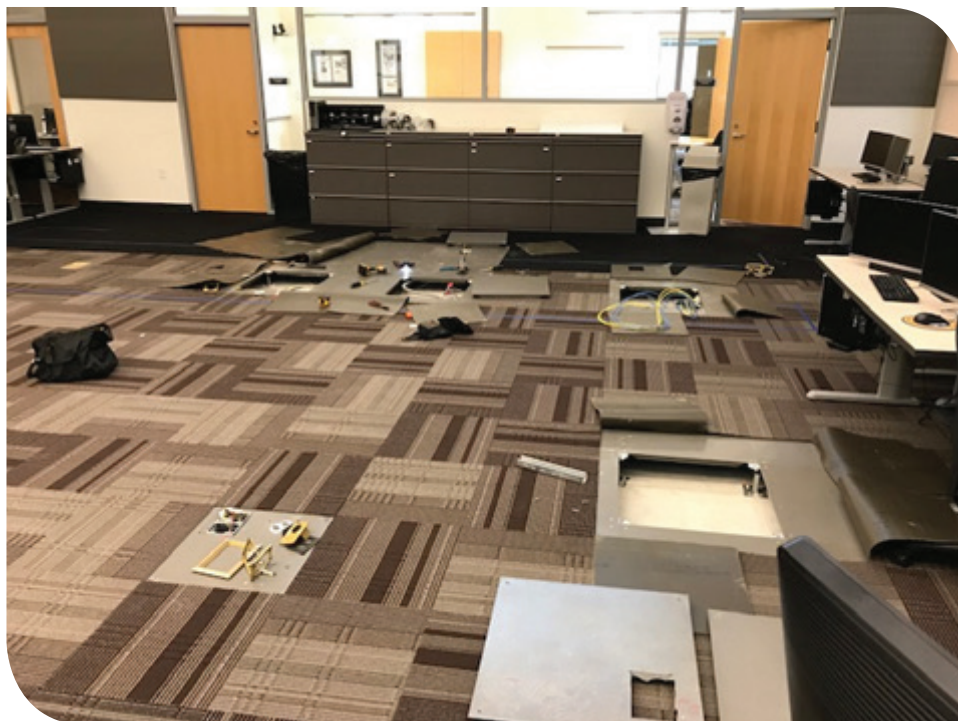
EOC electrical work
