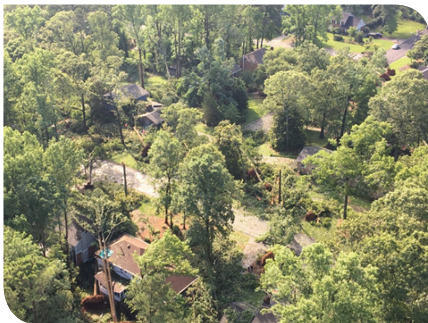
June 1 downburst damage viewed from AIR1
